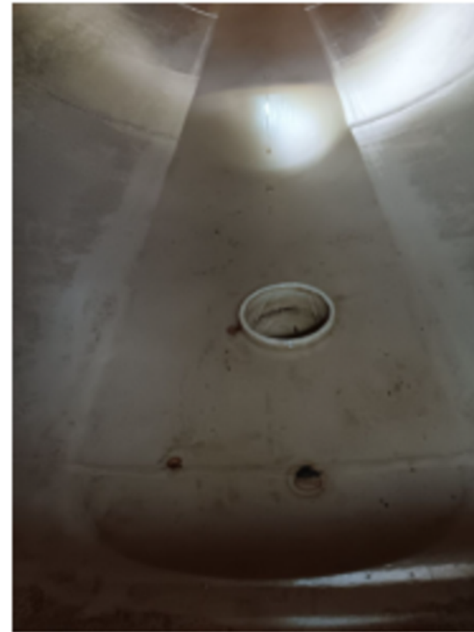
Pressure Tanks After Cleaning
